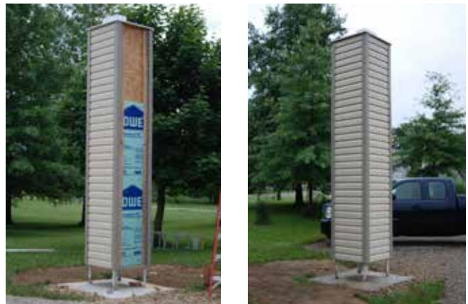
Left: A “Gray’s Anatomy” shot with the cap section on the top and painted, one side finished, the other side edged, insulation in the bottom of the side (an 8’ tall section of insulation) and the wood showing at the top. Insulation was added there before siding coverage.
