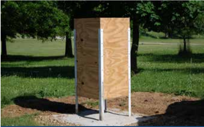
The base section with the concrete poured – a ton-plus of dry quick-crete mixed with water and added to the existing concrete.
